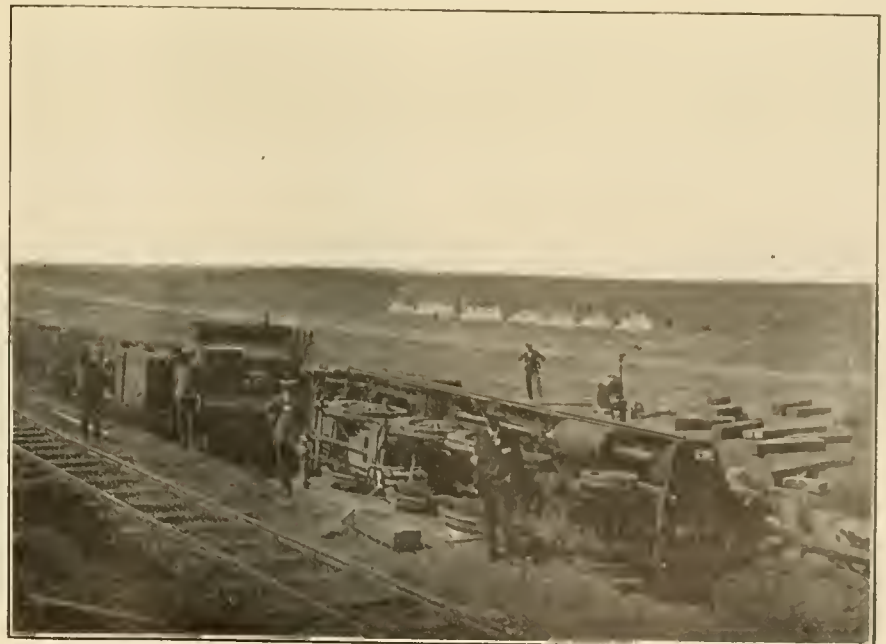
INCIDENT IN SOUTH AFRICAN WAR. RAIL REMOVED FROM TRACK.
